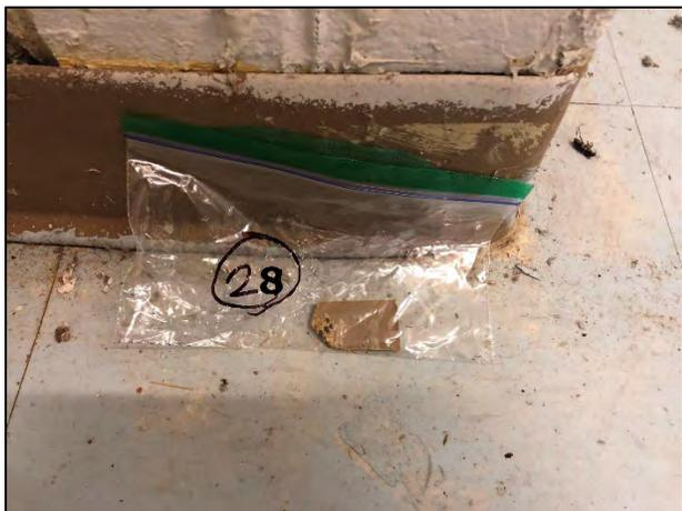
Sample #28-Asbestos containing cove base mastic
