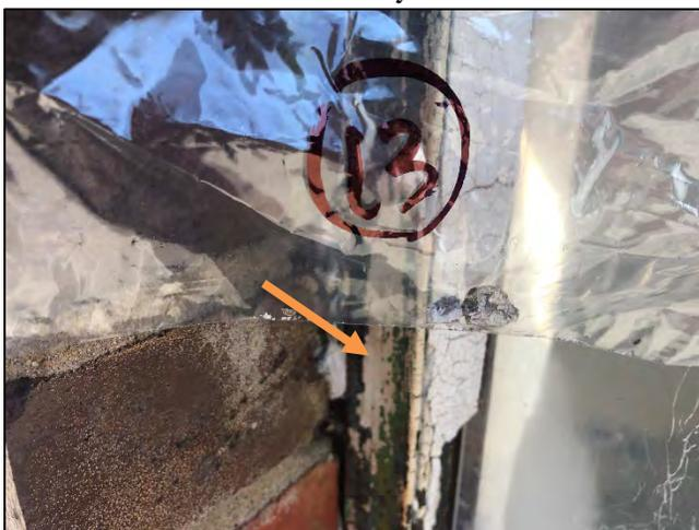
Sample #13-Asbestos containing exterior window caulk
