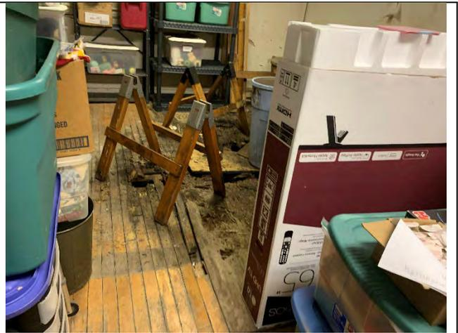
**Photo 6: extensive water damage in storage room 1**
