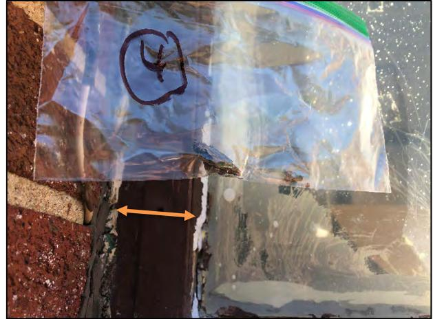
Sample #4-Asbestos containing exterior window caulk
