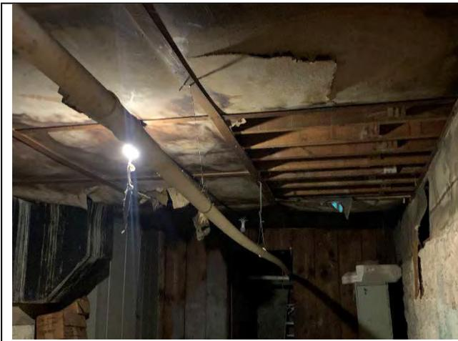
**Photo 3: water damage and suspect mold growth on the basement ceiling material**
