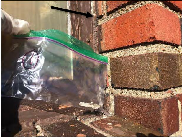
Sample #1-Asbestos containing exterior window caulk
