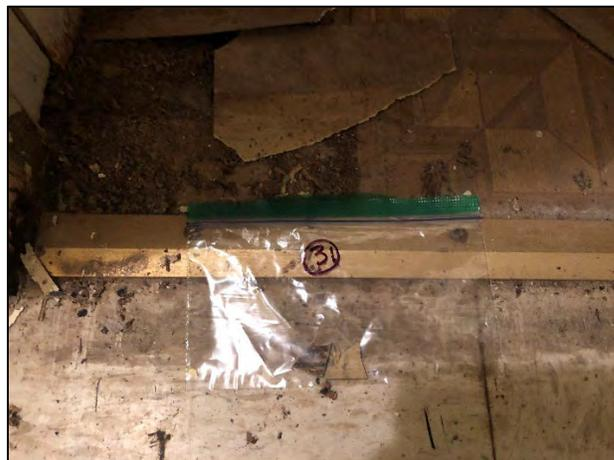
Sample #31-Asbestos containing floor mastic
