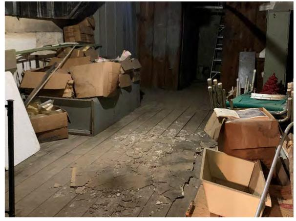
**Photo 2: strong moldy odor and signs of water damage in the basement. Porous items such as paper and cardboard should be disposed of**
