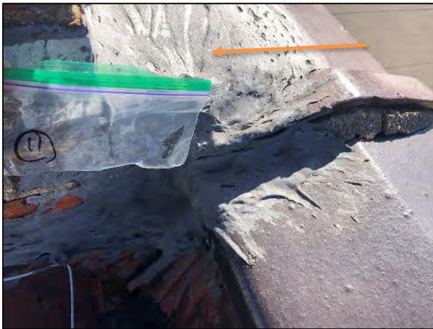
Sample #11-Asbestos containing roof patch at chimney
