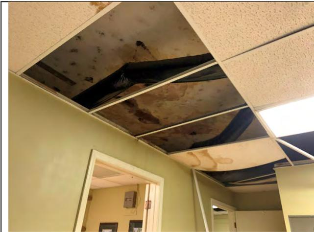
**Photo 5: water damage to the office ceiling**
